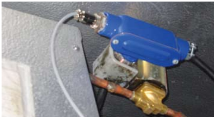
Photo 4: Signal Sensor Tee Installation
