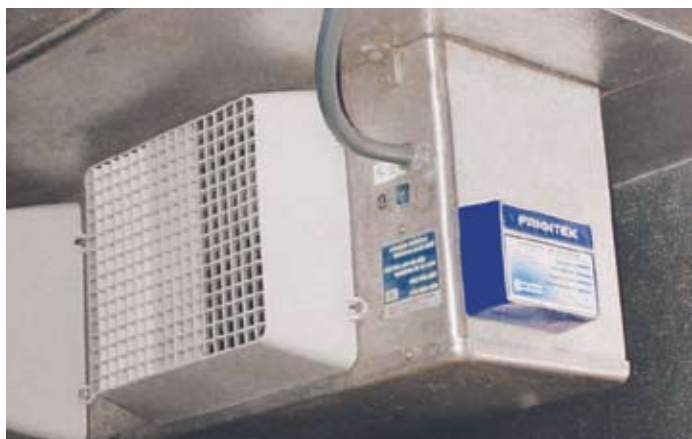
Photo 2: Evaporator Coil End Mount
